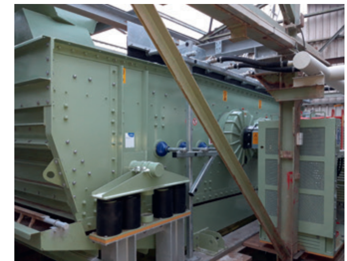
New Elliptical Screen (2,500 x 6,000 x 2) fitted into the existing steel construction
